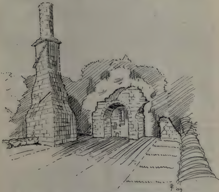
FIG. 65. ROOM OVER MUNIMENT ROOM.
